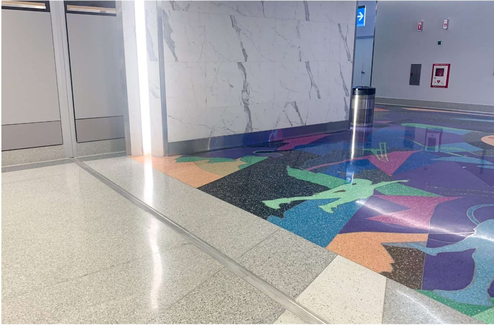
Single Interlocking Hinge Seismic System (SIH) inlaid with terrazzo floor (provided by others).
