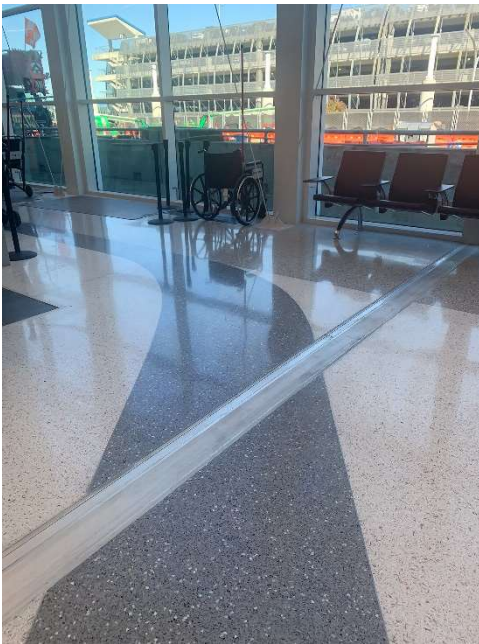
Dual Interlocking Hinge Seismic System (DIH) spans across the lobby inlaid with terrazzo floor (provided by others).
