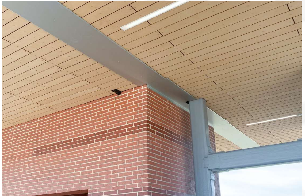
ASCL Expansion Joint Cover under the elevator awning.
