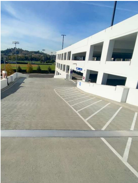
BIS installation on the parking deck ramp.
