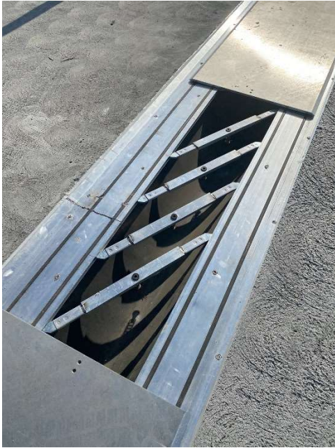
Customized Bolt-In Seismic System (BIS) at installation.
