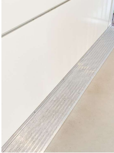
Hinged Safety Cover System (HCS) at the elevator core.
