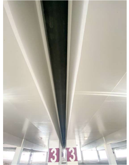
Flexible Rubber Gutter System (FGS) on the under-side of the BIS System installation.
